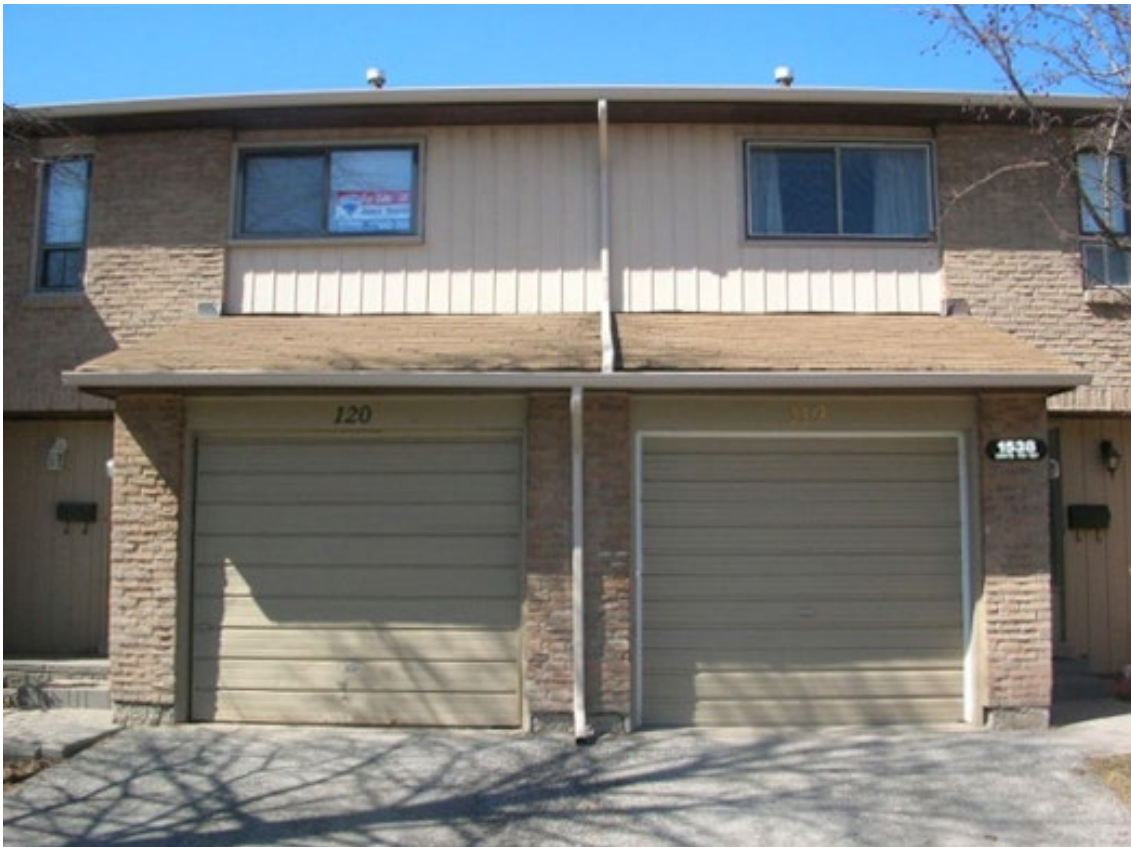
Use downspouts to direct water from upper to lower roofs; this reduces wear on the shingles.
