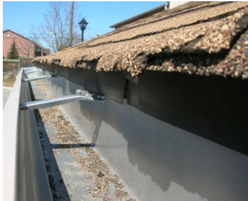
Aged shingles have ragged edges and lose their coloured granules (see debris in the gutters)
