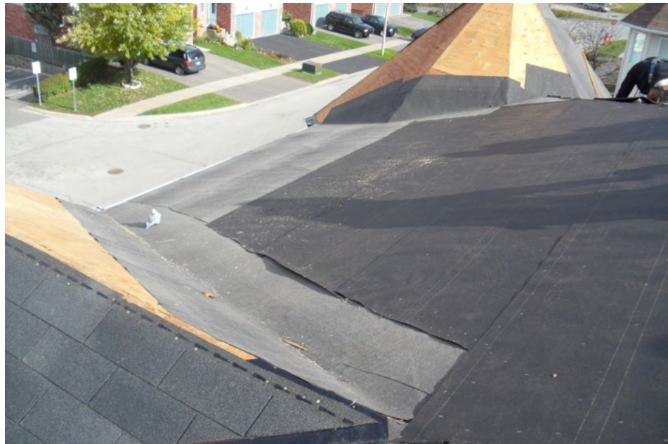
Waterproofing membrane (lighter grey) installed at base of roof and in valleys; roofing underlayment (black sheets) covers remaining plywood before the shingles are installed.
