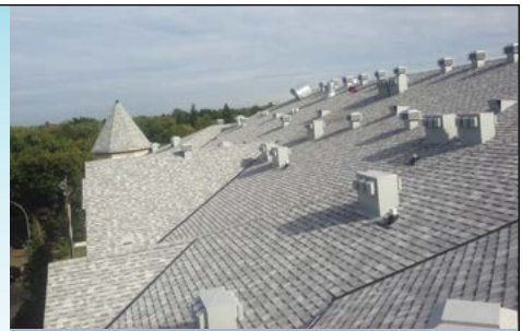
Commercial roof Asphalt Shingle Ventilation Maximum vents
