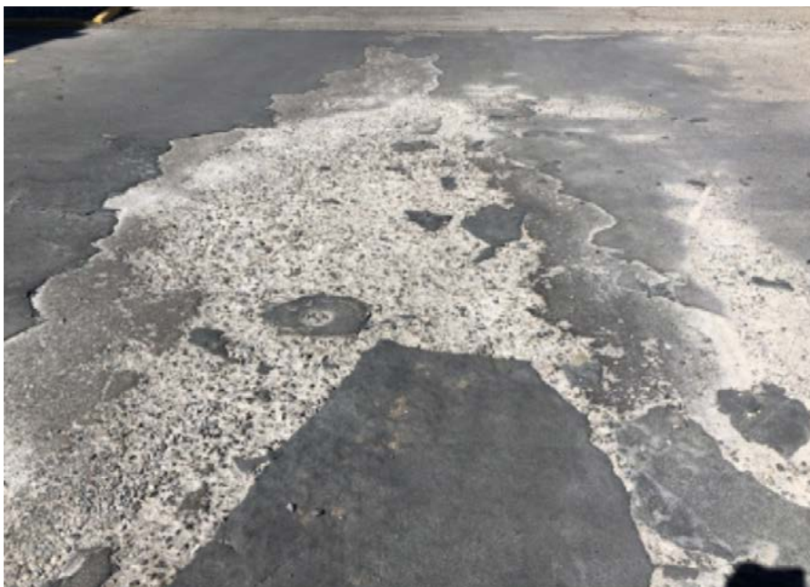
Figure 1 - Concrete Scaling due to Freeze Thaw
