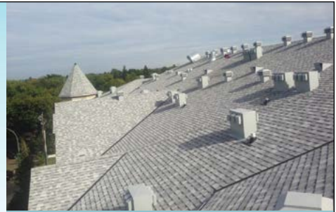
Commercial roof Asphalt Shingle Ventilation Maximum vents
